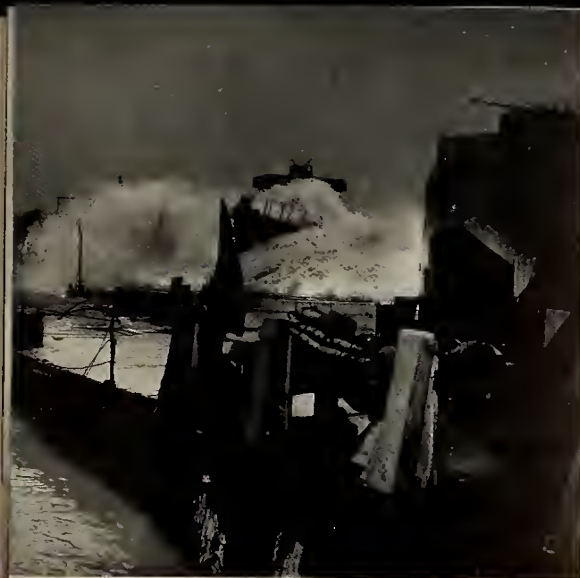
5. To supplement the caissons, sixty old Allied warships and merchant ships sailed under their own steam and were scuttled to form part of the breakwater. One of them was the old British warship, H.M.S. Centurion , shown above.
